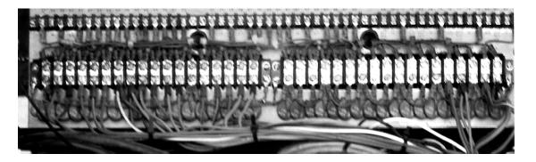
The field wires from the pedestrian and vehicular signal heads are attached to these terminals.
