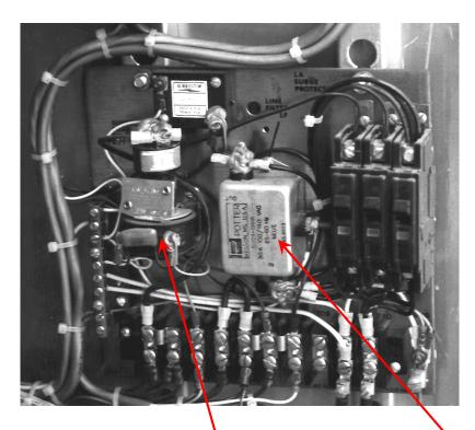
Before being fed to electrical devices within the cabinet, the electricity from the power company is passed through a <u>radio interference suppressor</u> and a <u>surge suppressor</u> that are located on the power panel. Also located on the power panel are a series of circuit-breakers which protect against current overload.
