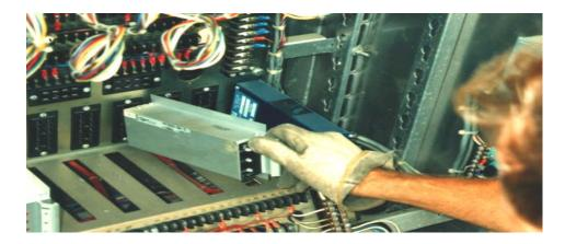
The load switch has 12 large male connectors that plug into 12-hole sockets located on the back panel of the controller cabinet. These sockets are commonly referred to as the load switch "bays".
