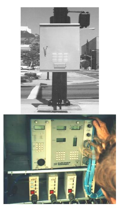
The field wires from a pole-mounted cabinet either run through the back of the cabinet to the center of the hollow support pole to which it is attached, or run through the bottom of the cabinet to steel conduit mounted on the outside of the support pole. Ground mounted cabinets are typically bolted to a concrete foundation with the heads of the bolts set in the concrete and the cabinet attached to the concrete using a set of washers and nuts.
