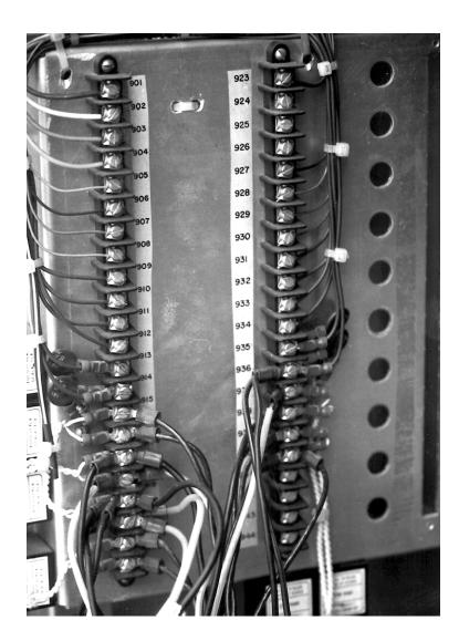
The field wires from the inductance loops are attached to terminals located on the detector panel. In many cabinets, field wires from the pedestrian detectors are also terminated on this panel.
