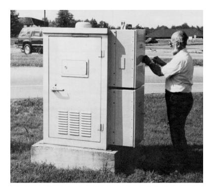
With the widespread use of low-power-consuming LED traffic signal displays, and with the increasing power storage capabilities of modern batteries, the capability to run signalized intersections for extended periods of time on batteries alone has been constantly improving. In fact, it is getting to the point where charging these new batteries using solar or wind power is a feasible way to power an entire signalized intersection on a permanent basis; not just as a back-up plan.
