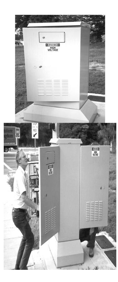
A slot within the Type 170 controller is reserved for a standardized Prom Module which contains the software used to control the Type 170 system. The inputs and outputs controlled by this software are highly flexible and logic can be written into the software to control devices other than standard traffic signals. Ramp metering signals, changeable message signs, uniform sprinkler system, can all be controlled using a Type 170 system with the proper software.
