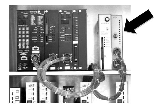
If the conflict monitor detects that two conflicting phases (phases that control conflicting vehicle movements) are active at the same time, the monitor will immediately place the intersection into latched flashing operation. A phase is considered to be active if it has either a green, yellow, or walk indication. Latched flashing operation is flashing operation that will continue until the conflict monitor's reset button is activated.
